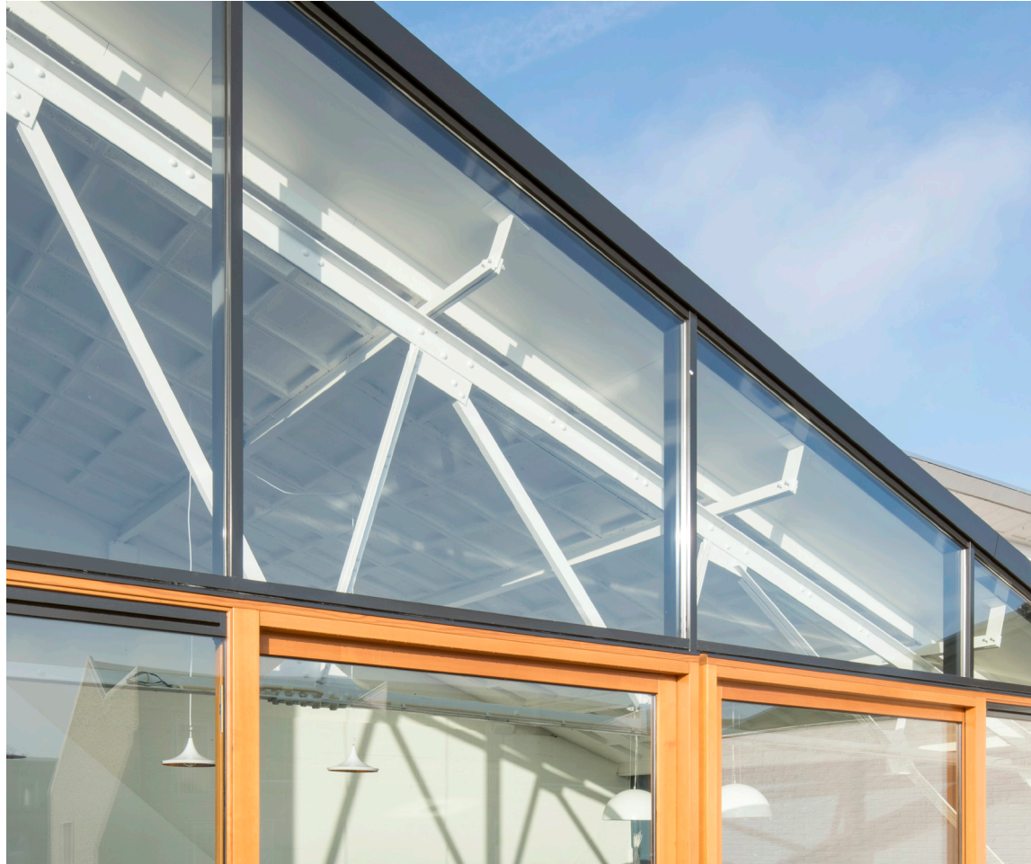
existing joists and the new facade
